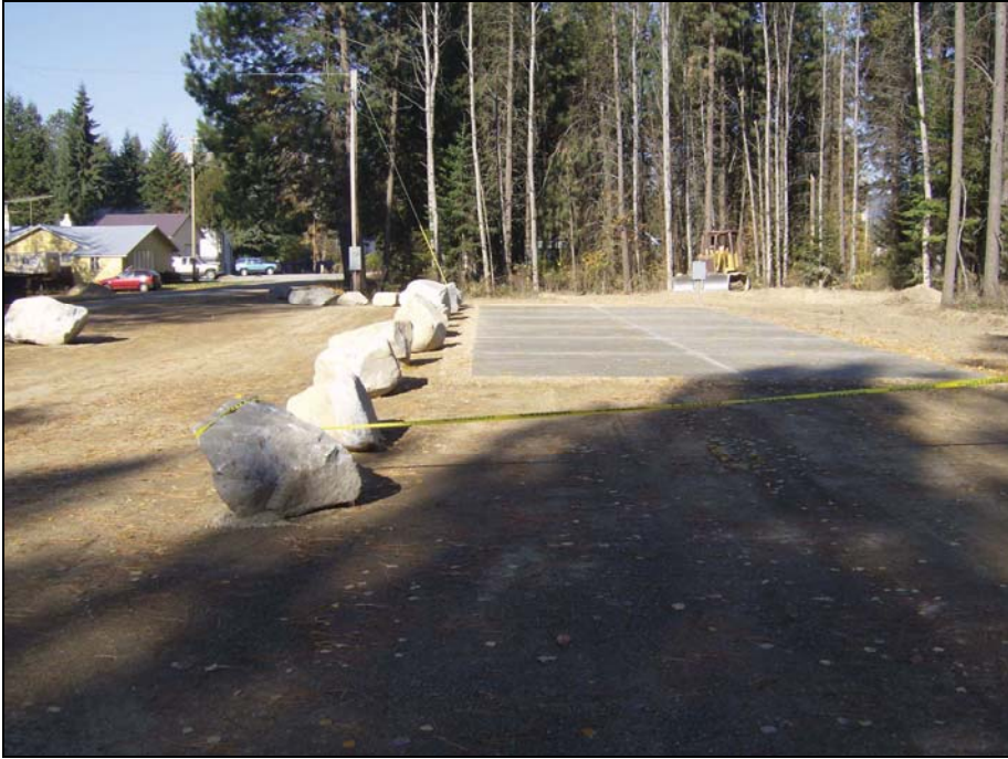
Sportsman Access Lake Host Facility Constructed As Part of Phase II
